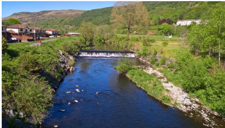
b) Merthyr Vale Weir - May 2018
