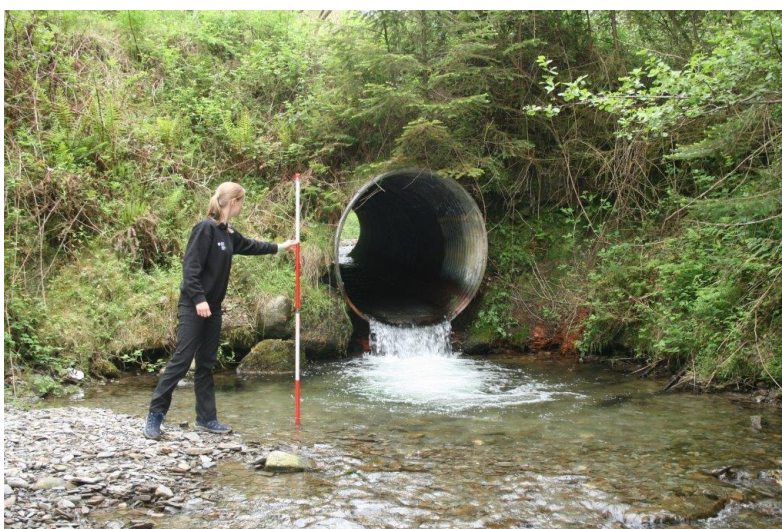
d) Typical forestry track culvert, pre-remediation, showing constraint to free fish passage
