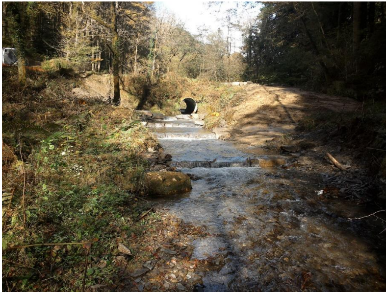
e) Forestry culvert post-remediation
