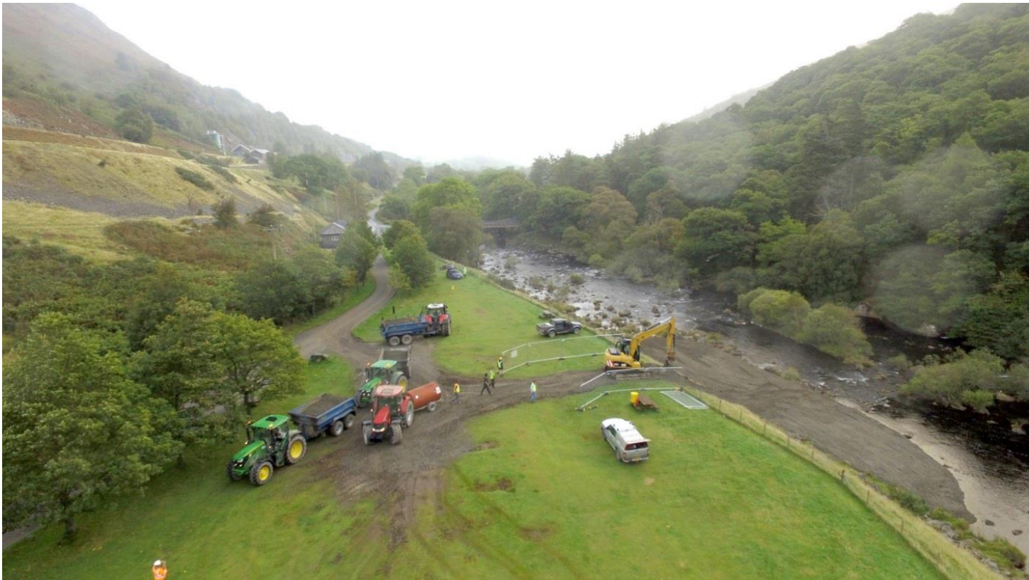
Figure 8: At Site 4 a platform was created with the first loads of gravel from which the remaining loads could be placed into the river channel
