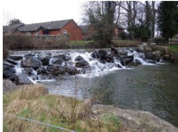
The weir at Kington: note the raised crest with vertical sides. This has enabled most of the flow to be directed via a leat to a turbine
