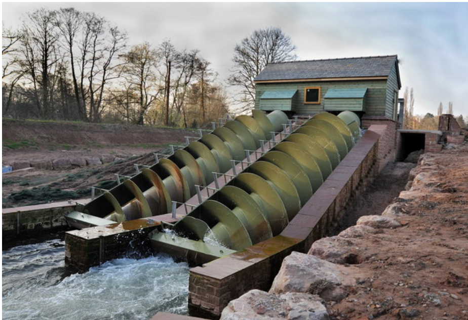
Above – The Osbaston weir hydropower station on the Monnow
